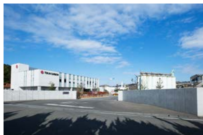
Expansion of CIP material production capacity at Tanoura Plant in Kumamoto Prefecture
