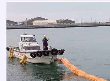
▲ Oil fence deployment for oil spill prevention (Ishinomaki Plant)
